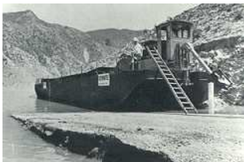
Dump barges' operation. A dump barge before launching.
