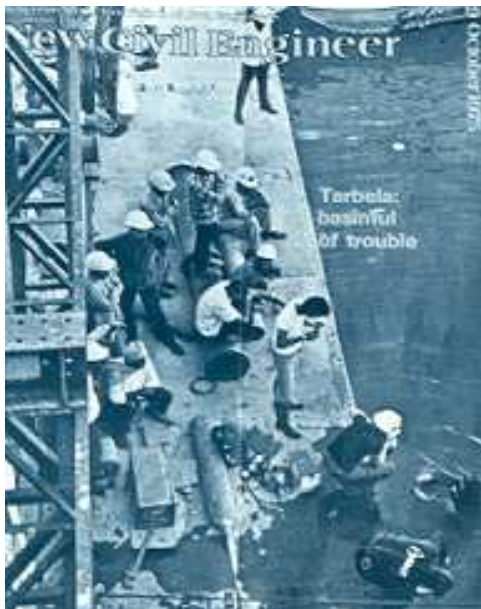
Stilling basins. Tunnel 3. Cover picture of the NEW CIVIL ENGINEER of October 9.75, showing the tremie concrete pontoon, and Sinmast Divers at work.
