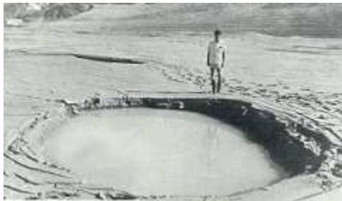
Impervious blanket. Typical sinkhole. (Oct.74)
