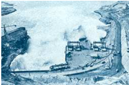
Outlet area. The drawdown. (Courtesy of Water Power and Dam Construction – June-July 1975)
