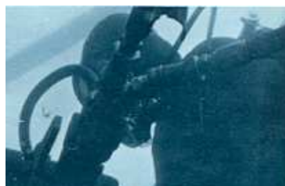
Intake tunnel 2. Installation of an hydraulic actuators system.
