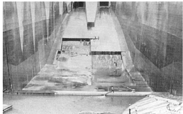
Stilling basins. Tunnel 3. After dewatering on summer 76
