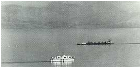
Dump barges' operation. The survey boat and a dump barge playing the Tarbela reservoir.
