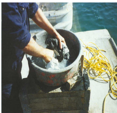
Hand mixing of the 2 components SUBCOM T.260.
