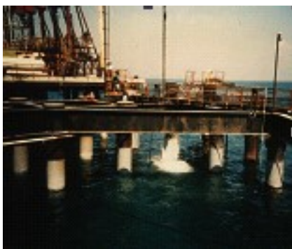
Underwater and splash zone grit-blasting.
