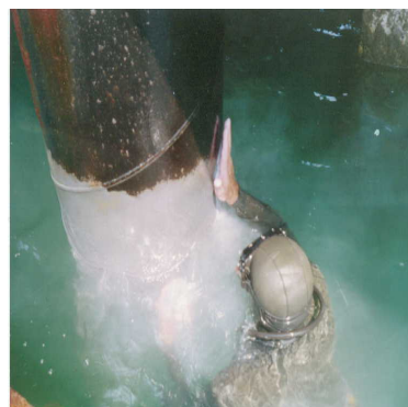
Application by manual spreading of SUBCOM T.260.
