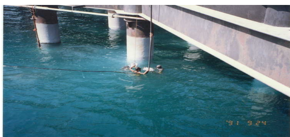
Application by manual spreading of SUBCOM T.260.
