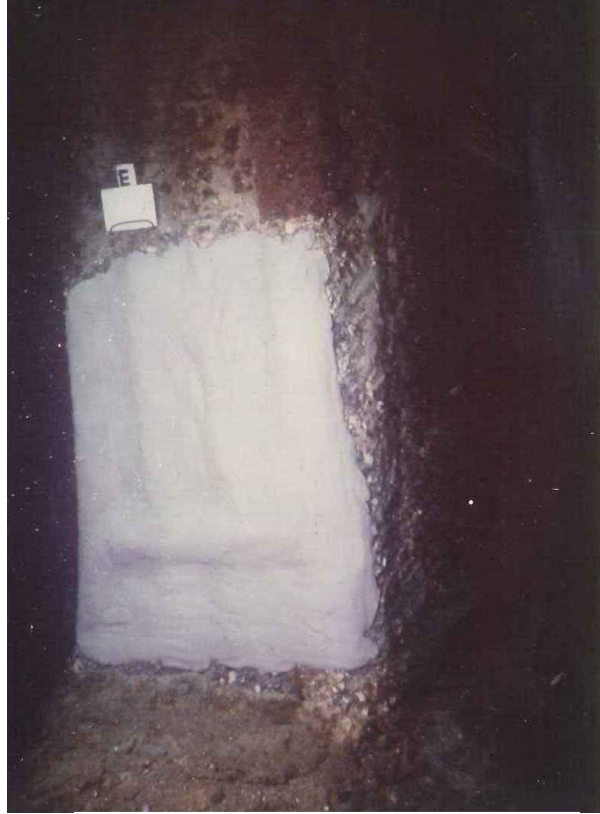
Underwater exposed reinforcement protected with SUBCOM T.260
