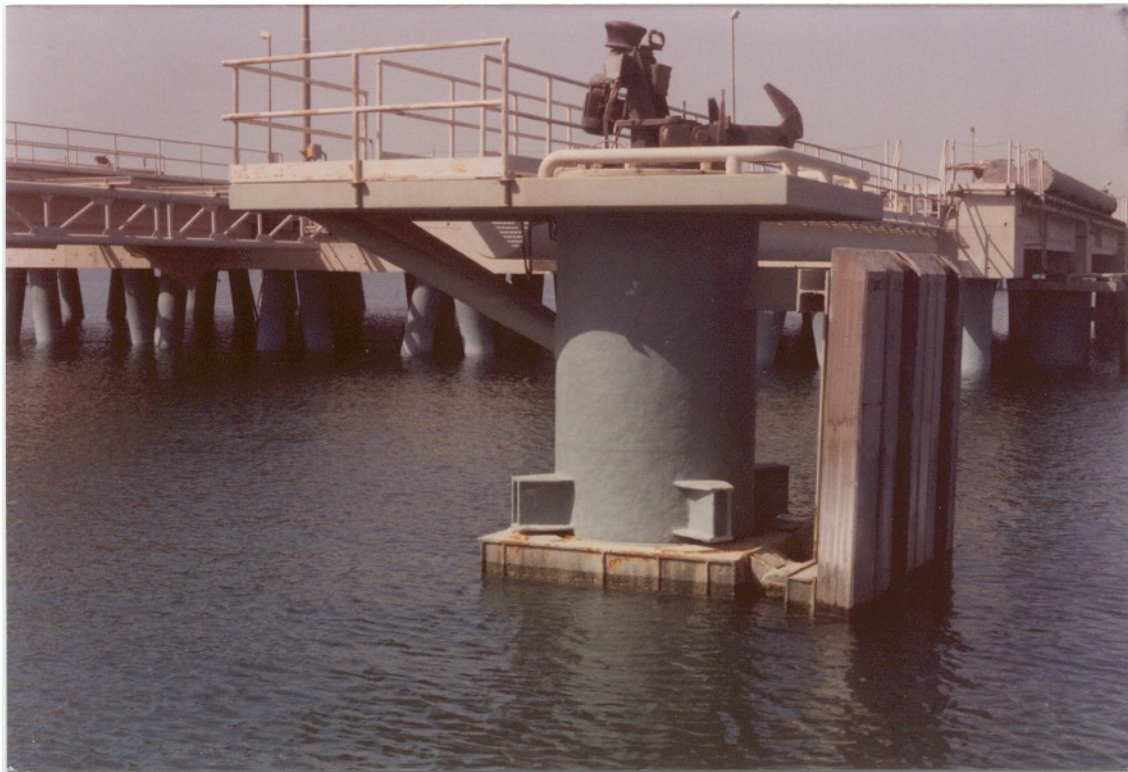
SUBCOM T.260 on jetty steel piles
