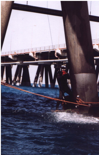
Grit blasting of splash zone
