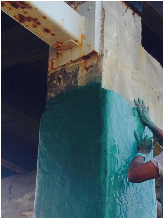
Application of SUBCOM T.260 on concrete piles
